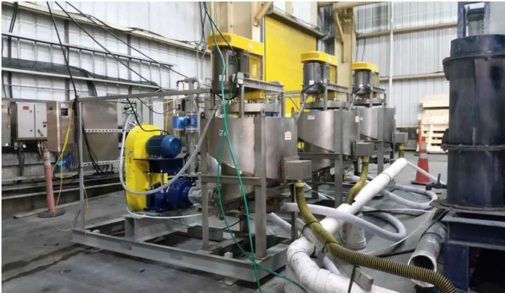
Figure 3: The train of three 0.61 metre diameter StackCells used in this pilot study.
